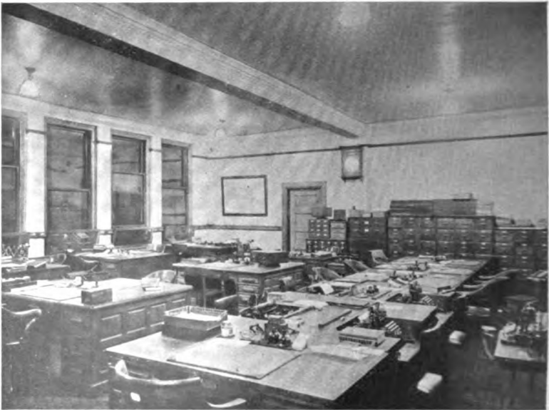
Section of Carnegie Steel Company's Offices, Pittsburg, Pa.—Correct Desk Lighting Effected by Holophane Shades Placed on the Ceiling, Giving a Uniform Light Distribution on Desk Tops, Causing Locally Arranged Desk-Lighting Units to be Unnecessary.
